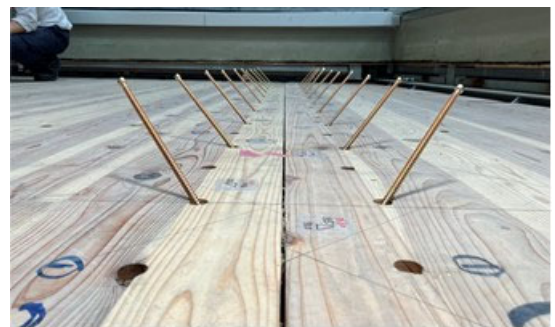
写真-1 立体的斜めビス接合の施工の様子 Photo.1 Installation process of a three-dimensional inclined screw joint
