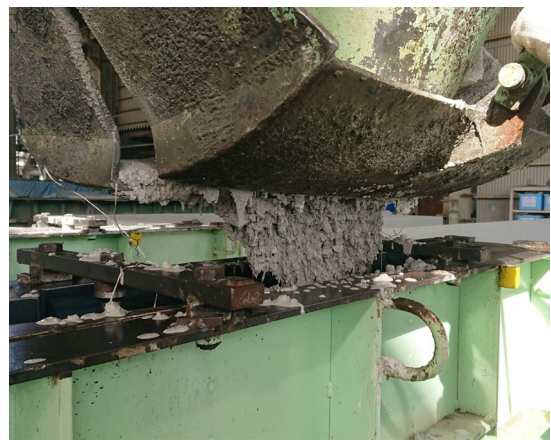
写真-6 Carbon-Recycle の打込み状況 Photo.6 Carbon -Recycle casting
