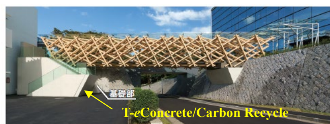
写真-2 Carbon-Recycle の現場設置状況 Photo.2 On-site application of carbon-recycle
