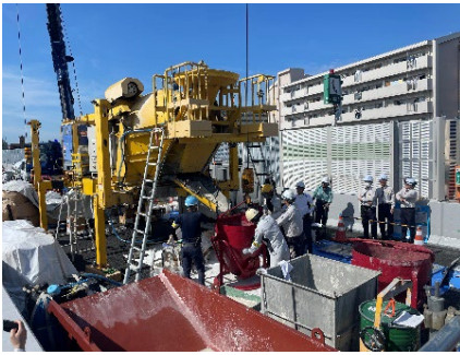
写真-2 練混ぜ Photo.2 Mixing
