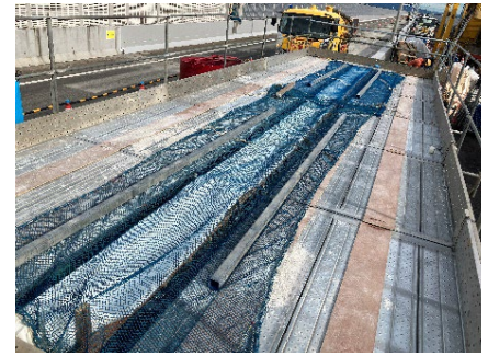
写真-4 湛水養生 Photo.4 Ponding curing
