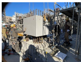
写真-2 壁脚接合部 PCa 部材形状および取り付け状況 Photo.2 Shape of Pre-Cast member of wall bottom joint and its installation
