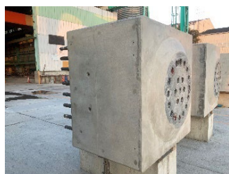
写真-2 壁脚接合部 PCa 部材形状および取り付け状況 Photo.2 Shape of Pre-Cast member of wall bottom joint and its installation
