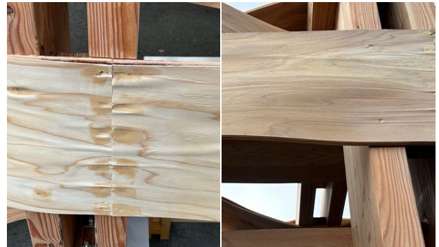
(a) 表層の波打ち・割れ (b) 部材の膨潤 (a) Rippling and cracking of surface (b) Swelling of the component
