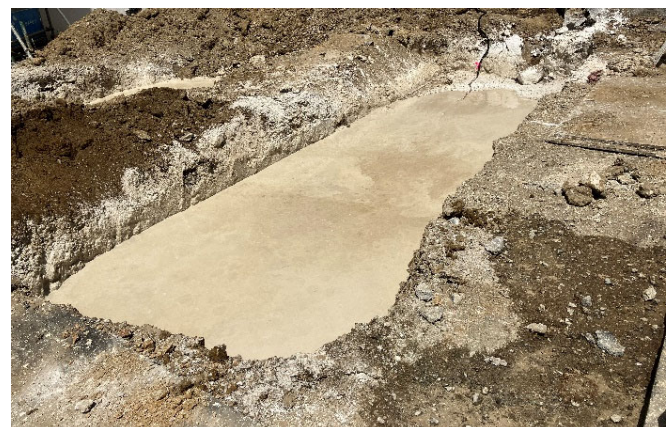
写真-4 施工完了状況 Photo.4 Completed improved ground
