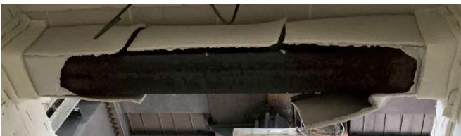
写真-2 加熱後の試験体 Photo.2 specimen after heating
