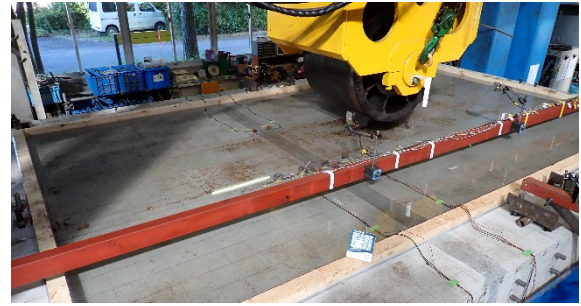
写真-5 漏水確認試験の状況 Photo.5 Water leakage confirmation test
