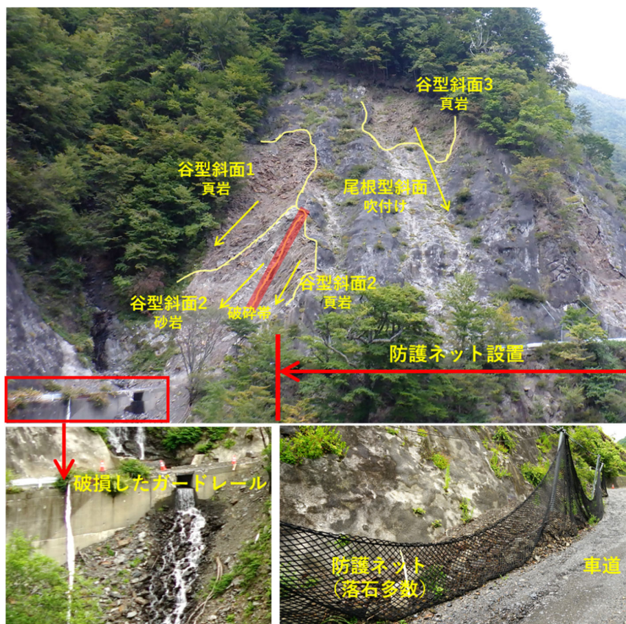
写真-2 落石監視を実施した斜面の状況 Photo 2 Slopes where rockfalls were monitored
