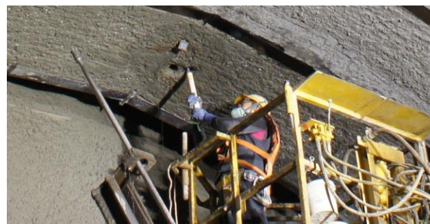
写真-4 天端傾斜計の設置 Photo.4 Installation of the inclinometer
