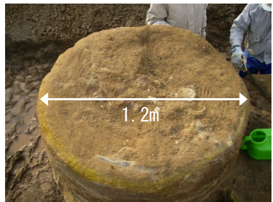
写真-3 改良体の造成状況 Photo.3 Observed solidified body (artificial ground)
