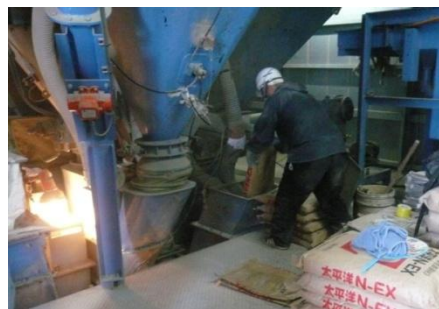
写真-4 早強性膨張材の投入 Photo.4 Put into high-early expansive additive
