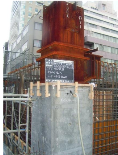
写真-5 下階柱とパネル間の目地グラウト充填 Photo.5 Grouting of seam between lower column and panel
