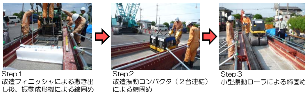
図-22 実験 (その 2) 状況 (Step1~Step3) Fig. 22 Experimental compaction Part 2 from Step 1 to Step 3
