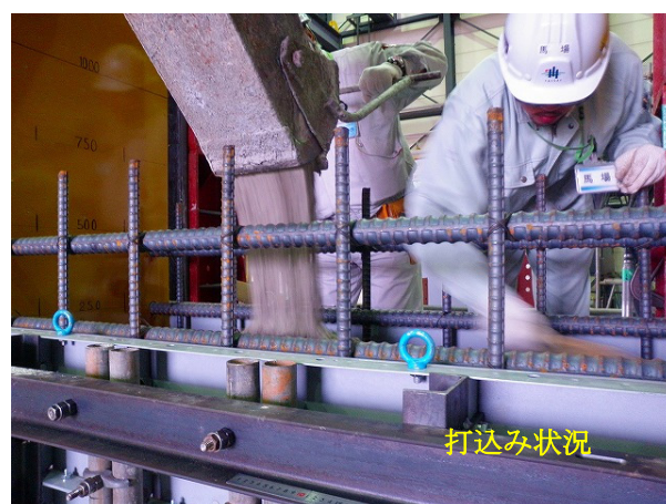
写真-1 打設状況 Photo 1 Casting condition
