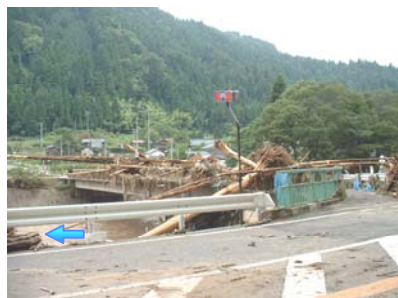
写真-1 橋を乗り越えた流木 Photo.1 Driftwood which got over the bridge
