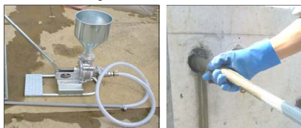
図-7 モルタルの充てん Fig.7 Filled by mortar
