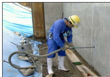
図-5 孔内清掃 Fig.5 Cleaning of holes
