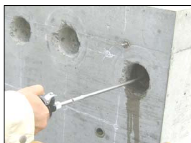
図-6 孔内湿潤 Fig.6 Humidification of holes
