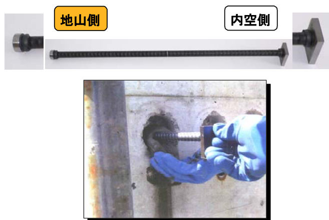
図-8 Post-Head-barの挿入
