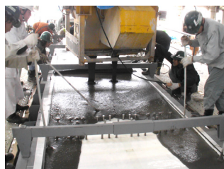
写真-7 U桁打設状況 Photo 7 Casting of Ductal
