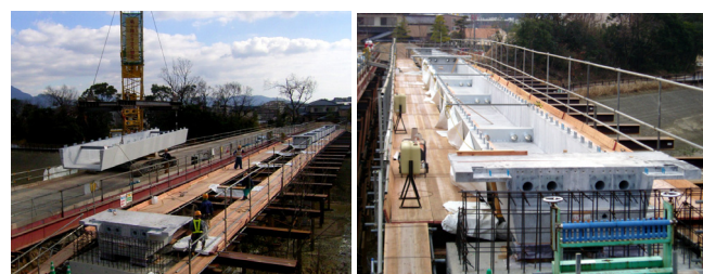
写真-10 U桁架設状況 Photo 10 Erection of U-shape girder
