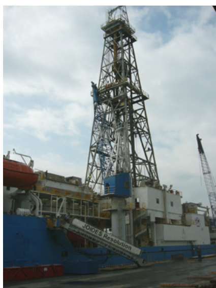
写真-8 船中央に立つ掘削用檣 Drilling Scaffold in Center of the Ship
