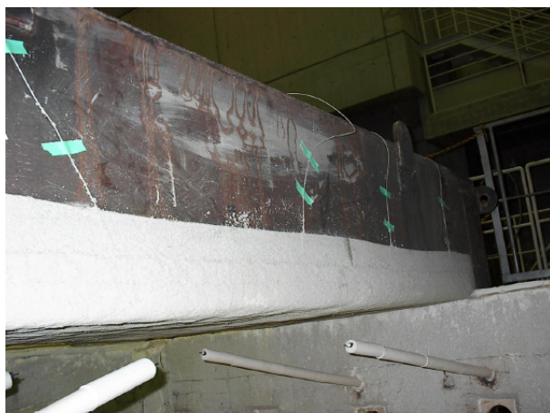
写真-2 炉内温度測定用熱電対設置状況 Thermo-couples to monitor furnace temperatures
