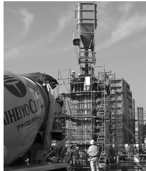
写真-2 1階柱の打設状況 Placing of concrete of column
