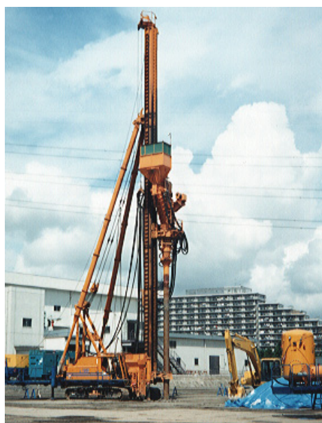
写真-1 静的締固め工法(SAVE工法) Non-vibratory Compaction Method
