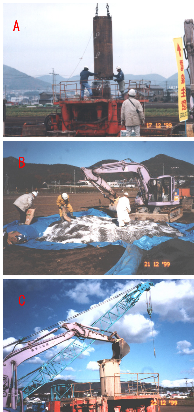
図-4 浄化壁施工状況 (A:掘削, B:反応剤混合, C:反応剤投入) Construction of the barrier (A:digging, B:mixing of materials, C:inputting materials)
