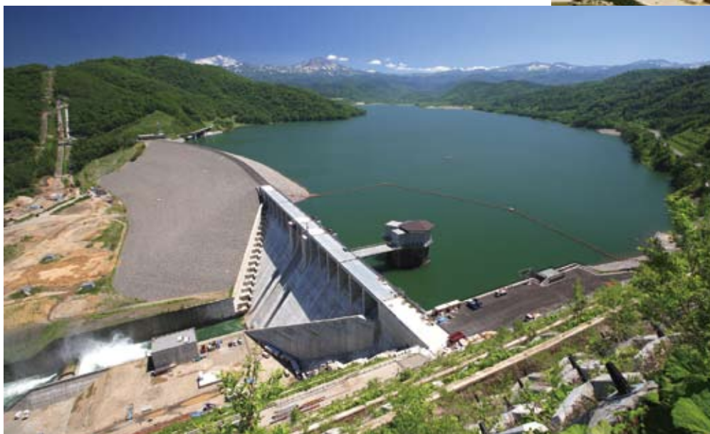
Chubetsu Multi-Purpose Dam Project, Construction of Rock-Fill-Dam (Phase V) (Hokkaido, Japan)
