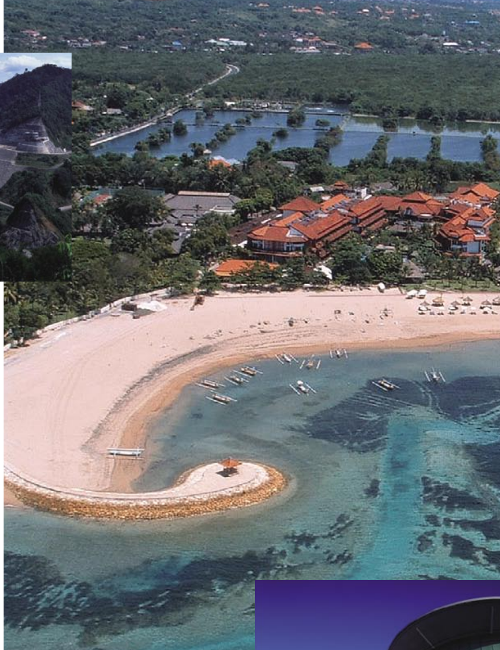
Bali Beach Conservation Project, Indonesia
