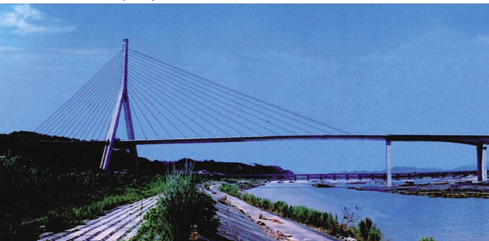
The 2,617m, six-lane Kao Ping Hsi Bridge, Taiwan
