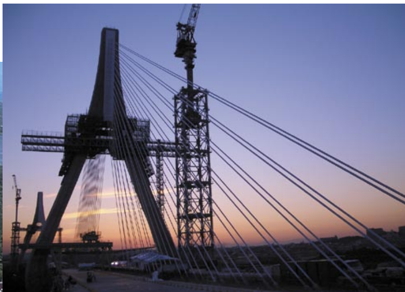
Yahagi Bridge, Japan
