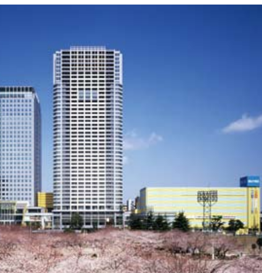
(Provisional name) Taihei 4-chome, Kinshi-cho Development Plan, Administration and Commerce Building (Tokyo, Japan)
