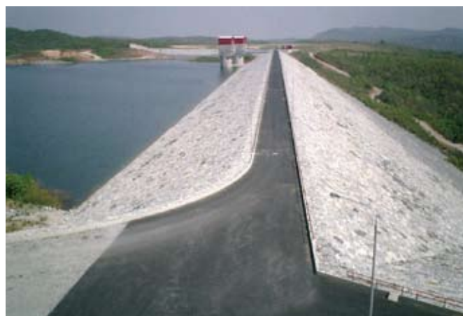
Purulia Pumped Storage Project Lot 4 - Main Civil Works (India)
